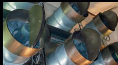
The continuous monitoring of the thermal load in the system enables the intelligent control of the number of active fans, the air speed, and the air volume. When the demand drops, entire air cooling units are switched off and actively defrosted.
